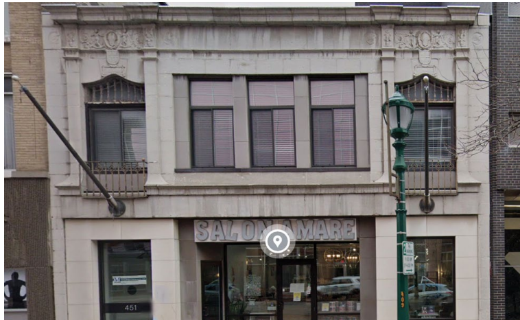
Existing Exterior Front View (Front Facade)
