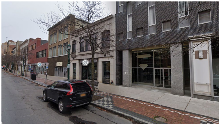
Existing Exterior Side View (Front Facade)
