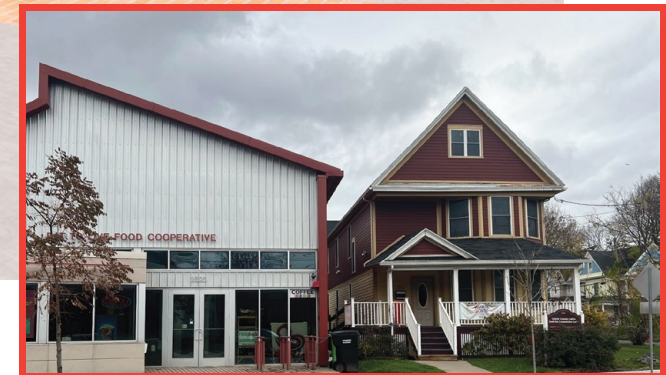
Existing (Current) Condition of the Site. 2331 S Salina St, Syracuse, New York 13202
